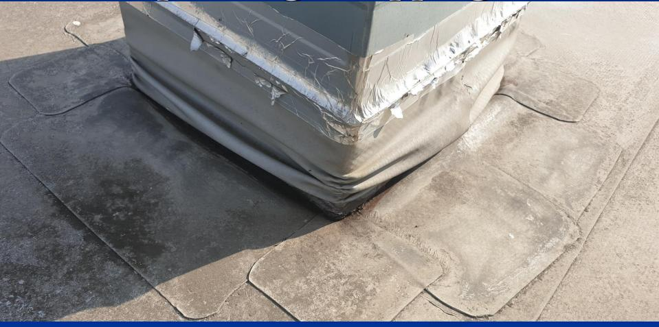
Very complicated details that can only be solved with liquid-applied waterproofing, e.g. PMMA
