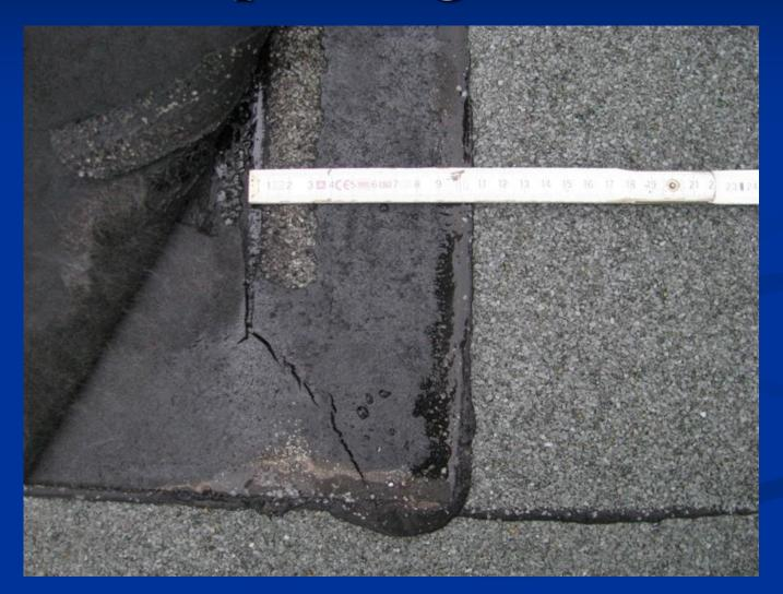
Delamination of bitumen waterproofing materiál, absence of asphalt penetration of the reinforcement
