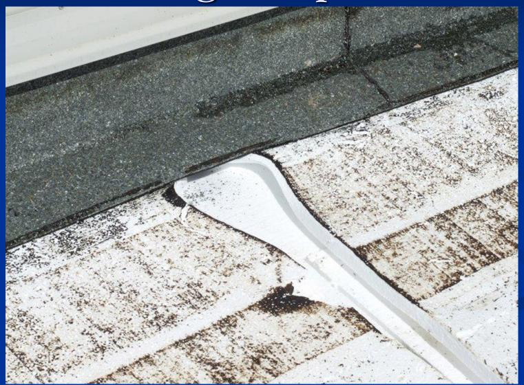
Degradation of the strength of mineral fiber thermal insulation due to heavy traffic
